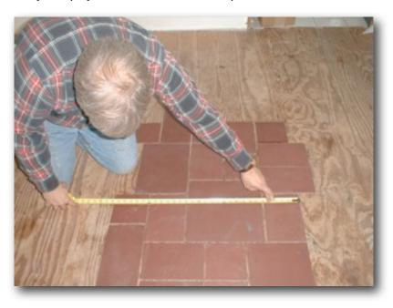
following the illustration on the box of slate. The critical part of this step is to ensure that the pattern itself is square. In my case, I started laying the slate tiles on the floor along a straight seam in the plywood flooring. The line of the pattern I chose was the one across from me where you see the end of the tape measure. Three of the five tiles in the pattern align on that line, the only two being the 9x9 slates that overhang the seam in the plywood.
