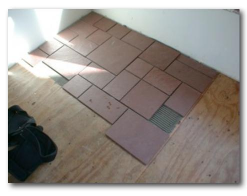
I've repeated the photo here again to point out another important thing you need to do. Since the slate is being installed along straight lines and the edge of the slate pattern is not straight because of the odd-shaped pieces of slate, you sometimes have thinset spread where you don't
