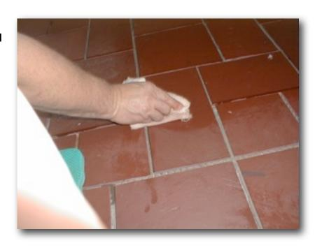
In this photo you can see me applying the clear liquid release agent to the top surface of the slate. Remember, before you do this you MUST allow the thinset to cure 24 to 48 hours. If you walk, kneel or twist your feet/knees on an individual piece of slate, you can
