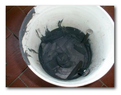
you added too much water. Water is a vital ingredient when mixing grout, but too much water when mixing, finishing or cleaning the grout will ruin it.
