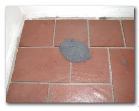
In this photo you can see I scooped out a glob of grout from the bucket. A 4-inch drywall taping knife is a great tool to use for this purpose. The grout you see in this photo is just about enough to fill the grout lines that are visible in the photo. You only want to apply as much grout as you can spread in an area about 2 feet by 2 feet square. You can
