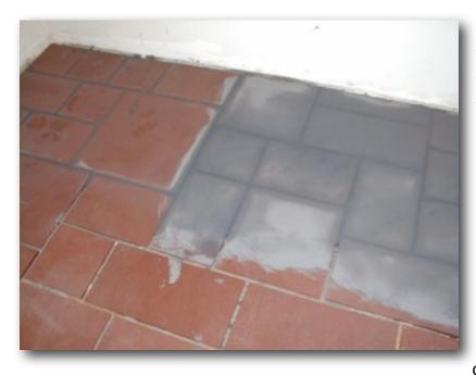
You can see in this photo that about 10 - 12 square feet has been grouted. Of that, about 4 square feet has been cleaned of the grout residue. The finished slate that's been grouted and cleaned is in the left side of the photo.
