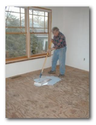
screwed it to the 3/4-inch Douglas-Fir plywood and then installed granite tile over it. So far the gypsum underlayment has done a superb job.
