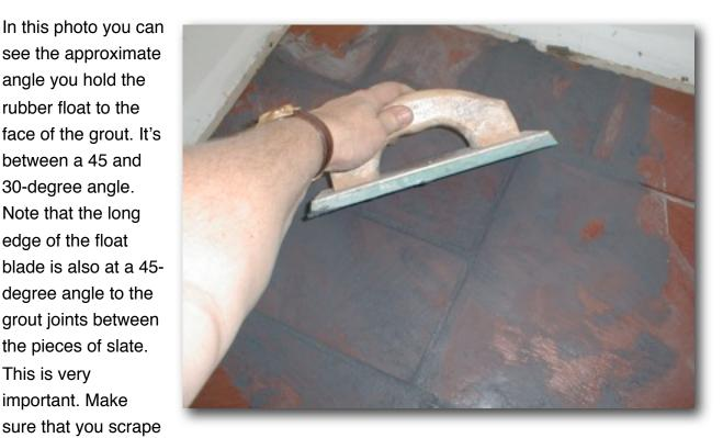
the float across the joints at this angle. Doing this prevents the edge of the float from dropping down into a grout joint and thus removing grout from the joint.
