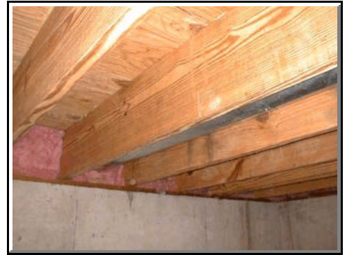
These are 2x12 floor joists under my own laundry room. They span approximately 16 feet and there is simply no bounce in that floor.
