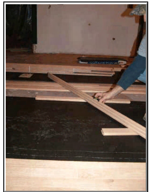
A straight piece of hardwood flooring can be used as a straightedge to find low spots in the subflooring. PHOTO CREDIT: Tim Carter
