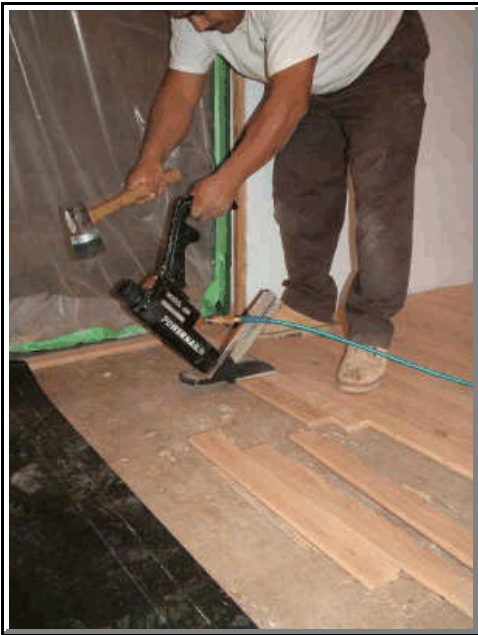
This air-powered nailer drives special nails through the tongue of the hardwood flooring. PHOTO CREDIT: Tim Carter
