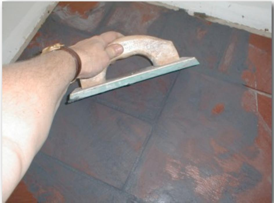
This is very important. Make sure that you scrape the float across the joints at this angle. Doing this prevents the edge of the float from dropping down into a grout joint and thus removing grout from the joint.
