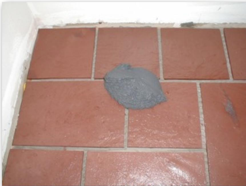
In this photo you can see I scooped out a glob of grout from the bucket. A 4-inch drywall taping knife is a great tool to use for this purpose. The grout you see in this photo is just about enough to fill the grout lines that are visible in the photo. You only want to apply as much grout as you can spread in an area about 2 feet by 2 feet square. You can
