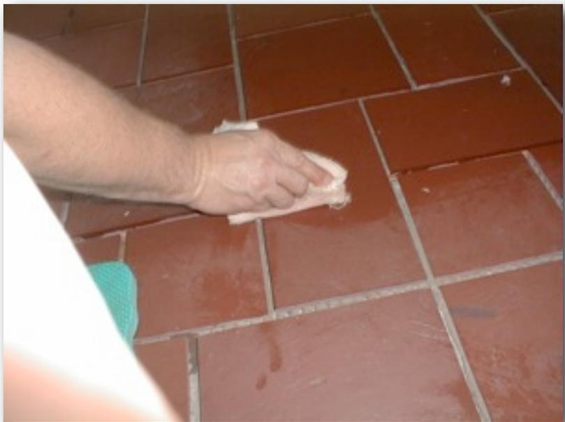
In this photo you can see me applying the clear liquid release agent to the top surface of the slate. Remember, before you do this you **MUST** allow the thinset to cure 24 to 48 hours. If you walk, kneel or twist your feet/knees on an individual piece of slate, you can
