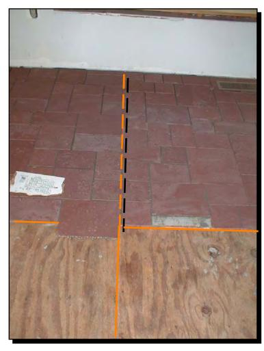
just too faint for you to see. The dashed orange line is the **center line** that's covered by the slate in place. The other chalk line that's in the photo is the second chalk line that is parallel with the original **base line**. The base line is already covered with slate in this photo.
