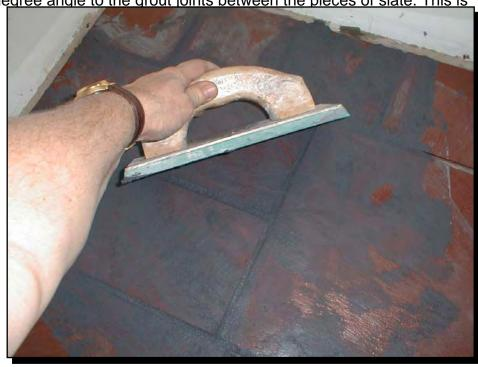
the top of the slate on either side of the joint. This will not always be easy as some slate can be thicker than others. You'll see how the rubber float controls this fairly well as you glide it across the slate.
