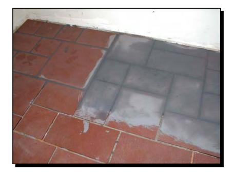
You can see in this photo that about 10 - 12 square feet has been grouted. Of that, about 4 square feet has been cleaned of the grout residue. The finished slate that's been grouted and cleaned is in the left side of the photo.
