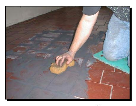
In this photo, you can clearly see that the grout haze is still going to be thick on the slate. In fact, there is still considerable grit from the silica sand on the face of each of the slate. That will be removed in the second step.
