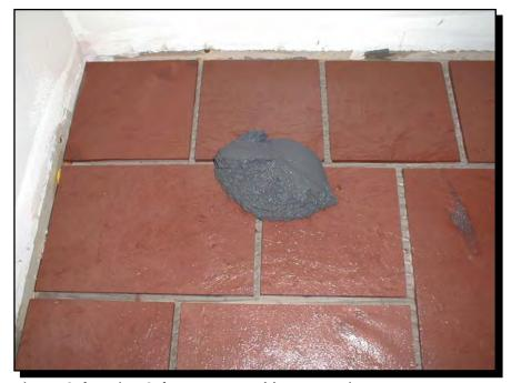
In this photo, you can see I scooped out a glob of grout from the bucket. Α 4-inch drywall taping knife is a great tool to use for this purpose. The grout you see in this photo is just about enough to fill the grout lines that are visible in the photo. You only want to apply as much grout as you can spread in an area
