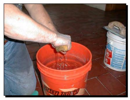
When you're doing this first phase of striking the joints, it's not so important to change the water frequently. The first time you rinse the sponge after rubbing it on the slate, you immediately soil an entire bucket of fresh water.
