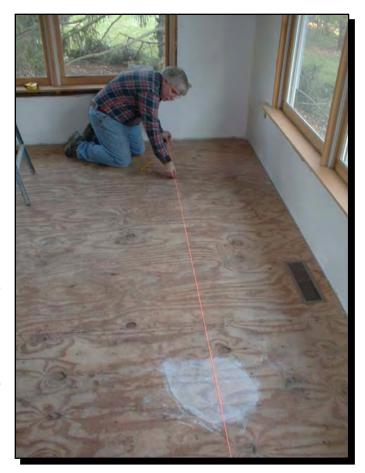
I use the chalk line to create this base line. Furthermore, I then snap a series of lines parallel with this one to keep my pattern in alignment. In my case, these lines would be 30 inches from each other as that accounts for the grout joint between each group of patterns. **Do NOT assume your pattern will work out to the same dimensions as mine.** You MUST do a dry layout of your slate to see what it works out to be.
