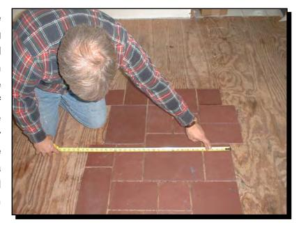
I chose was the one across from me where you see the end of the tape measure. Three of the five tiles in the pattern align on that line, the only two being the  $9 \times 9$  slates that overhang the seam in the plywood.
