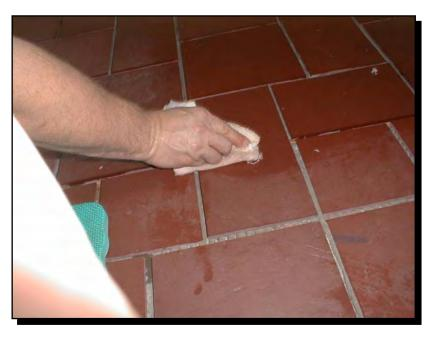
can break the bond with the thinset. Once the slate is grouted, it is much stronger and resistant to this damage as the grout interlocks all the pieces of slate into one giant slab.
