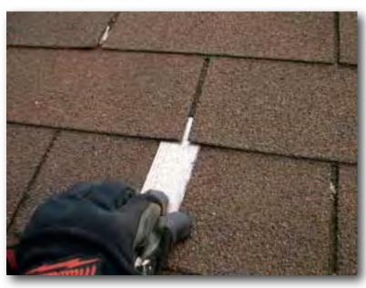
Here I am sliding the thin strip of metal up under the two tabs. You want to be really careful that you don't bend the metal putting a upwards hump in it or curling the bottom edge upwards. This will cause a hump in the shingle. You want the shingles to lay flat.
