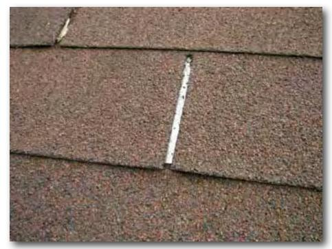
This is the finished look. The metal strip is in place, it's at the right height under the tab above and most importantly, the shingle tabs overlapping the metal to the right and left are smooth and flat.
