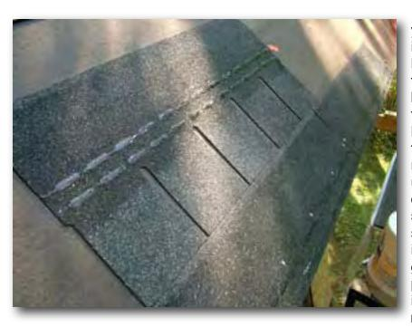
In this photo, I'm showing you an unusual shingle to illustrate what one looks like when you or a roofer takes it fresh out of a bundle. This shingle is a five-tab shingle made to look like a slate roof. See the five tabs? They are medium gray, and make up the lower 40 percent of the shingle. The shingle is resting on the starter strip of the roof so it wouldn't slide to the ground as I took the photo. I used these interesting shingles on my garden shed.
