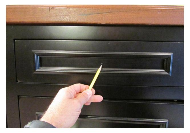
For repetitive holes in the same sized cabinets or doors, you can use a store bought drilling jig or a combination square set to the measurement you will be repeating. Use the combination square for drill hole marking.
