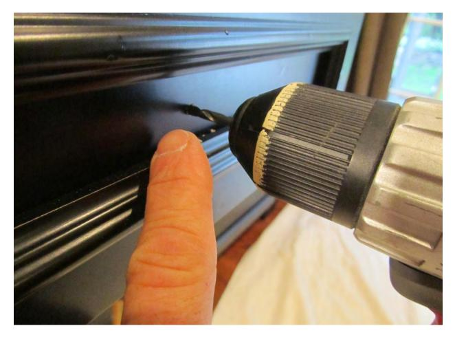
As you drill the hole through the door make sure to keep the drill perpendicular to the cabinet.
