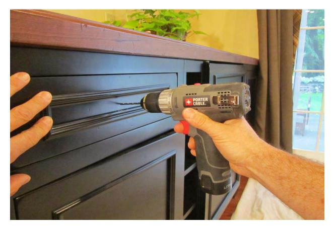
Be careful not to push the drill in too aggressively. You want to avoid the drill chuck from touching and damaging the finish on the cabinet face.
