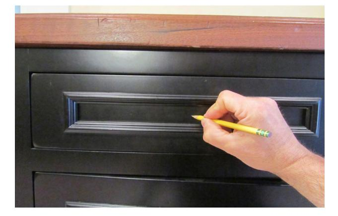
Mark the intersection of these two measurements with pencil and make a "+" mark.
