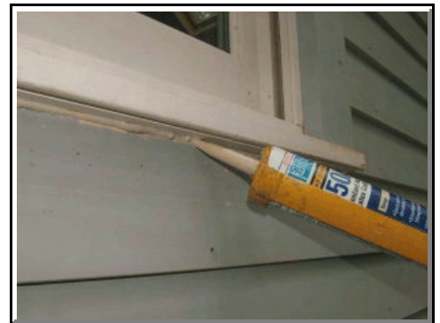
Caulk is a powerful weapon to stop water intrusion that can ruin a new house painting job. PHOTO CREDIT: Kathy Carter
